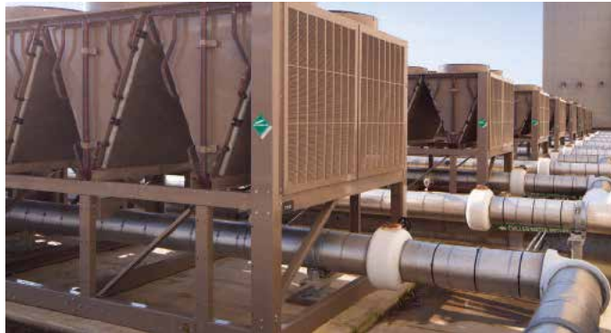
Closed-loop glycol only requires replacement every five years and there are no filters to change.
